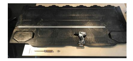
THE STEEL TUBES WE'RE AIMING FOR (underside of the deck) EASY MISTAKE # 2: Drill through both sides of steel tubes. <u>ONLY</u> drill through the top of steel tube
